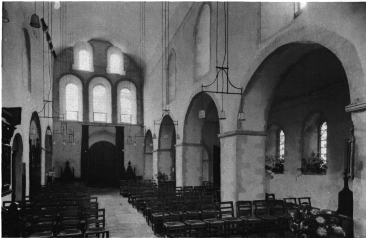
Interior of the Nave, looking West
