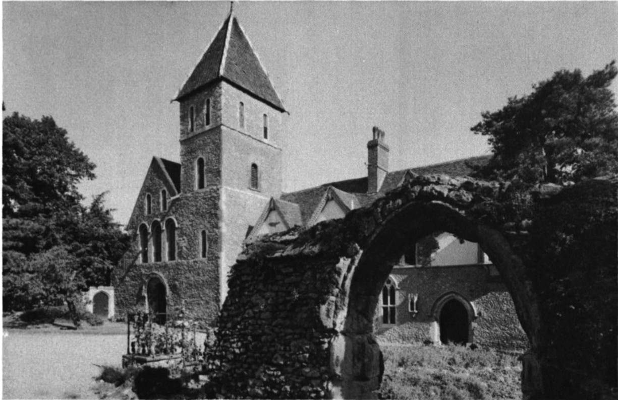
General View of the Priory from the South-West
